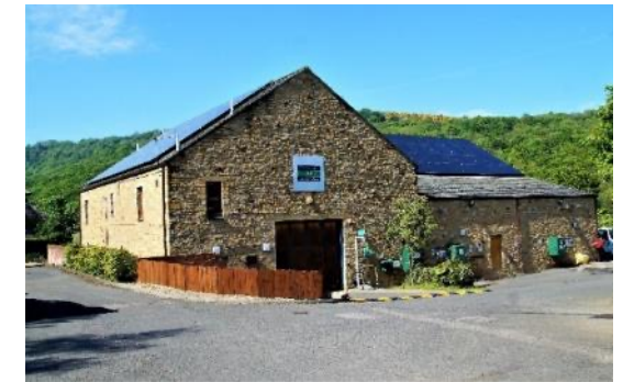
MOD Catterick: EV Rollout and PV Cells
